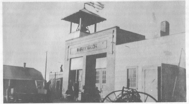
City Hall - 1916 - Blacksmith Shop
